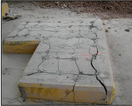
2. Breaking Reinforced Concrete, Cement, Rock, Limestone
