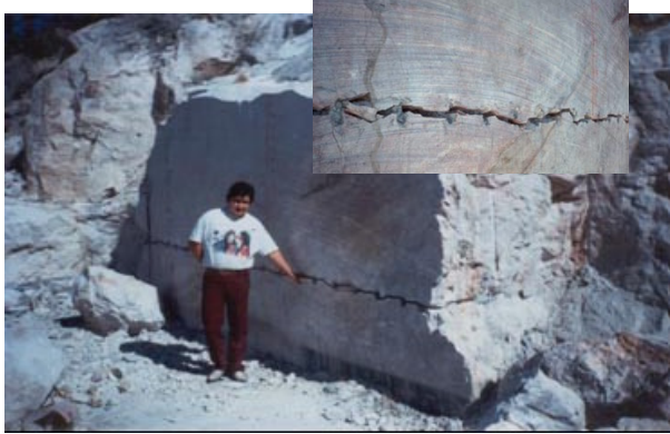
Non-Explosive Controlled Demolition
