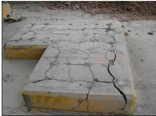
2. Breaking Reinforced Concrete, Cement, Rock, Limestone
