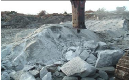
1. Demolition, Excavating, Remodeling Building Deconstruction
