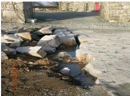
4. Other Demolition Work Where you can NOT use Explosives Or Traditional Equipment
